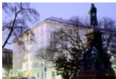
Outside View Schillerplatz
